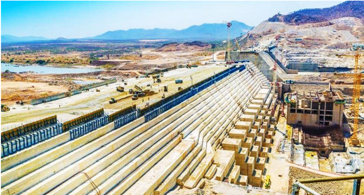
Overview of the construction of the Great Ethiopian Renaissance Dam (GERD)
